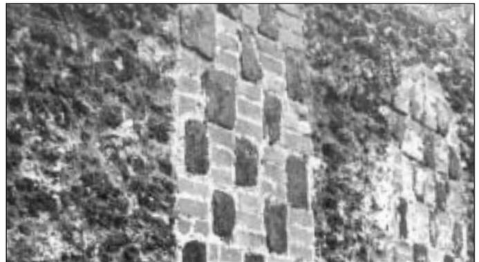
*Detail of Chequered Wall - showing a mix of brick, slag and clinker.*
