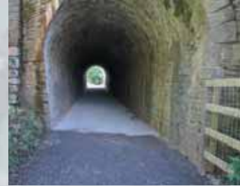
Carson's Road Tunnel
