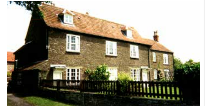
11 Old farmhouses are common features. Chestnut Farm at Mayshill, built from local pennant sandstone.
