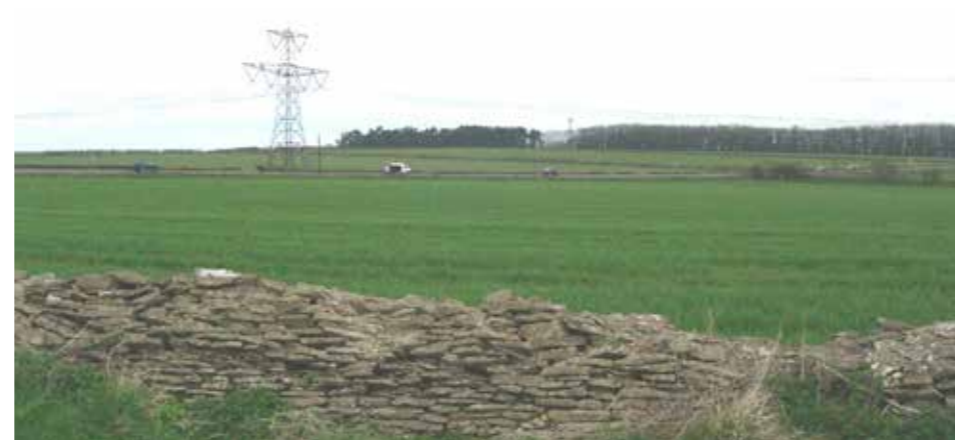
9 View towards the A46 and Beacon Lane Plantation. Pylon towers within this particular location are lower in height to limit the visual impact as they cross the skyline of the Cotswold Scarp.
