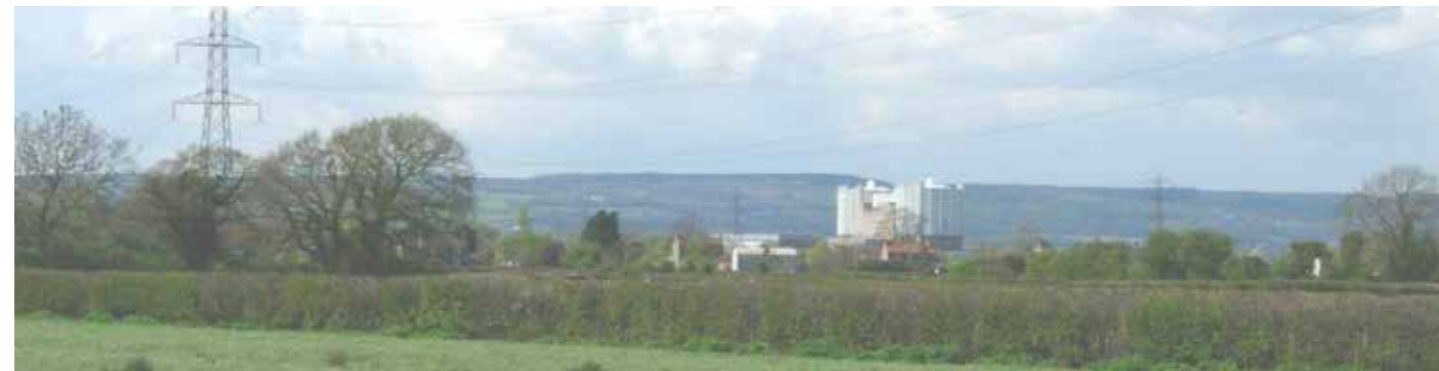
11 View towards Oldbury Power Station, with the farm buildings of Oldbury Naite in front and the Forest of Dean ridge behind.
