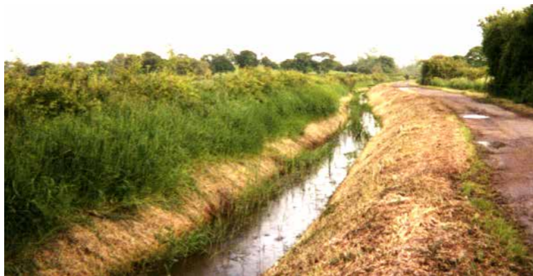
4 Deep drainage rhines are a characteristic feature with unmade road. Former marshland.
