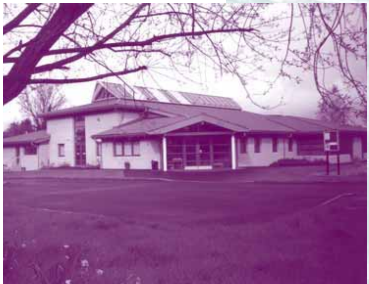
The new Manor School
