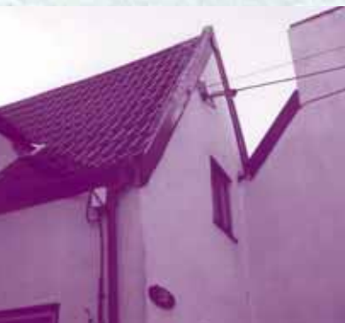
Woodend Road, Steep pitched roof.
