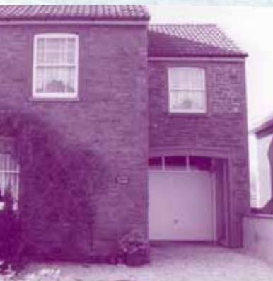
Extension built in sympathy with existing cottage, Henfield Road.
