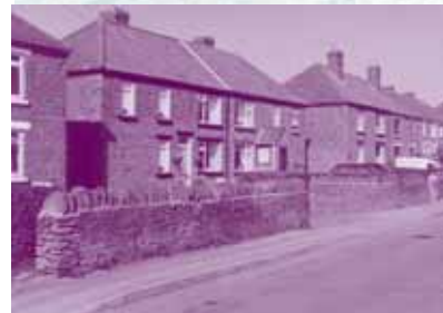
Local Authority built Wheatley Houses of unfussy design and proportion, Woodend Road.
