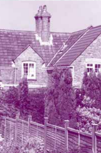
Rear of houses, Badminton Road Stonework, roof tiles and chimneys using characteristic materials.
