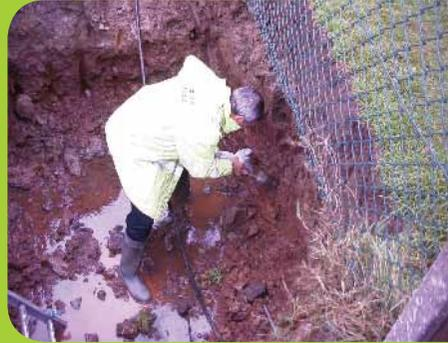
↑ Clean up of ground after leaking tank removed, showing drinking water pipe through ground.
