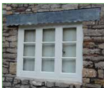
Traditional flush timber casement
