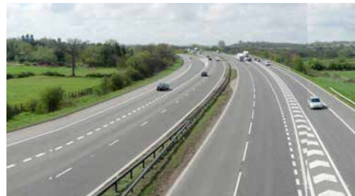
5 The M32 and broad largely green corridor, continues southwards to Bristol.
