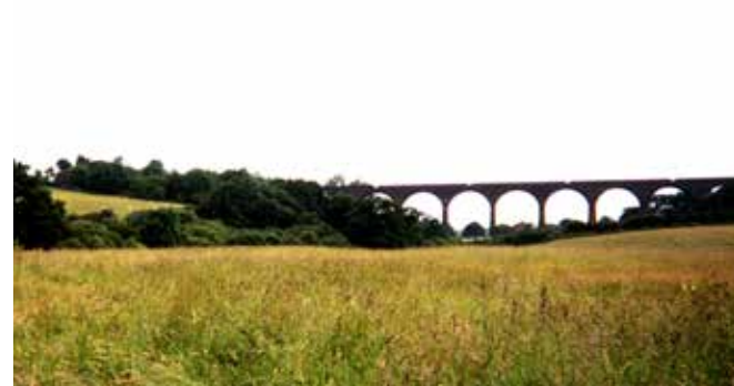
12 The River Frome valley and railway viaduct, looking northwards.
