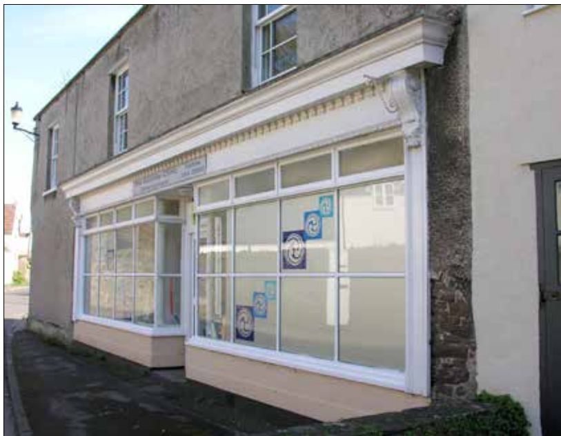
The ornate corbel brackets, fascia and cornice of a 19th century shopfront survive on this building in the High Street.
