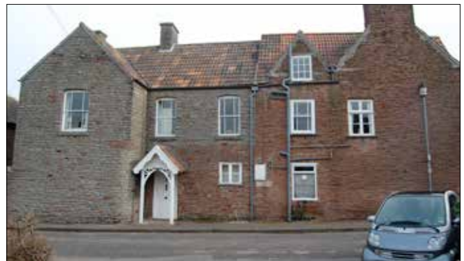
17th century The Gables with red and grey pennant stone showing different phases of construction.
