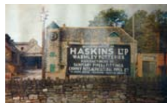
Clay pipe works, Warmley
