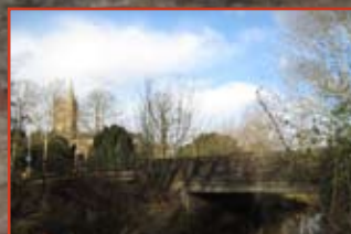
River Frome Bridge (7)
