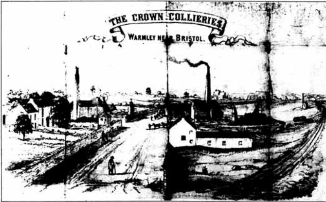
Crown Pit, Warmley—an old drawing thought to date from 1860. It shows the two main shafts each side of the road, both powered from the same engine house. The older pit standing close to the Dramway can be seen on the right of the picture. The engine house still stands but the chimney was demolished recently.
