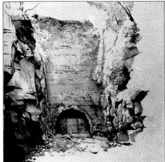
Wilsbridge Tunnel from the north.
