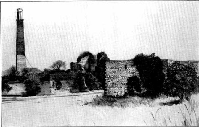
Brandy Bottom Colliery—remains of the horizontal engine house in the foreground and the older vertical engine house and the chimney behind.
